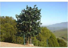
Figure 24 - An 'Elm' concealed cell phone tower manufactured by Valmont Structures
