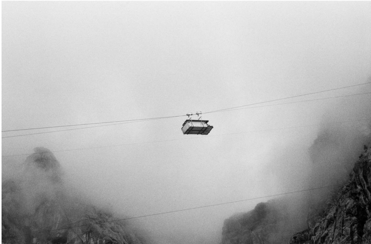
Figure 4: building materials being transported up by ropeway
