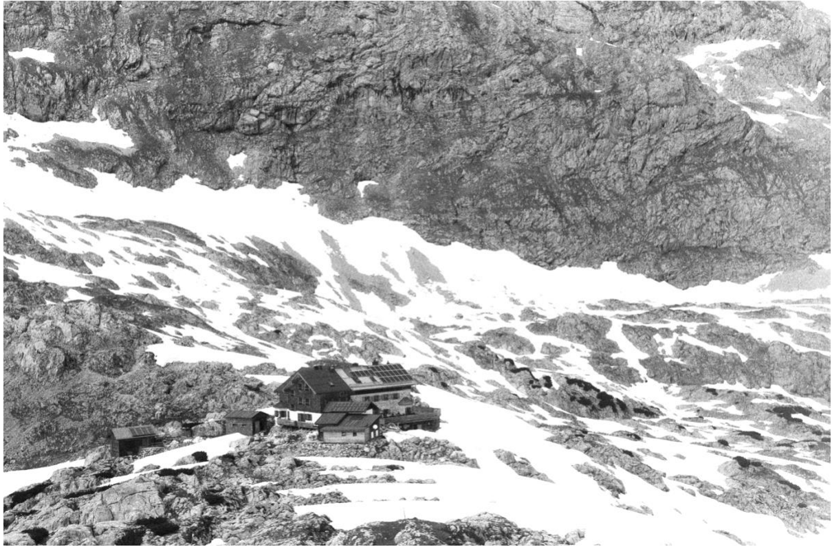
Figure 5: mountain hut with roof-mounted photovoltaic system
