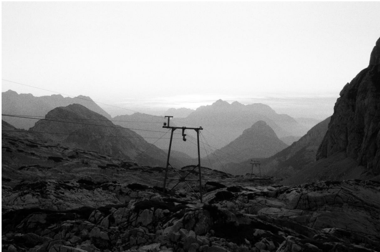
Figure 1: ropeway route to transport goods to a mountain hut
