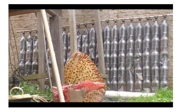
Figure 27 - The solar panel made of PET plastic bottles at Coopzumbi.
