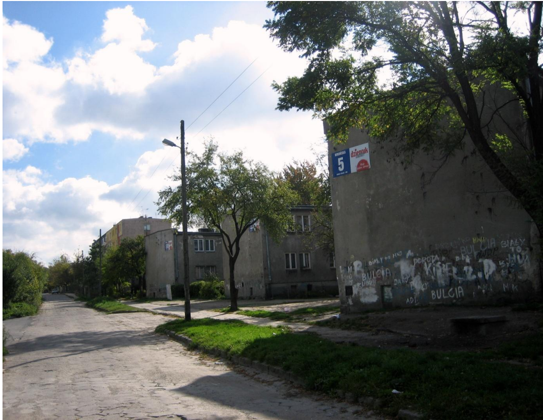
Figure 3 - Hotel Pumis (at the back) and three blocks of flats built during World War II for the purpose of accommodating concentration camp guards
