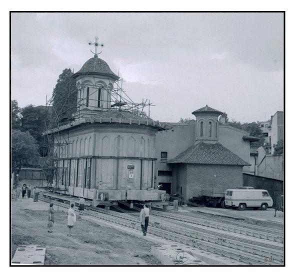
Image 33 - The small church is being moved to the new site, 200 meters away, documentation photograph. Source: <a href="https://www.rezistenta.net">www.rezistenta.net</a>.
