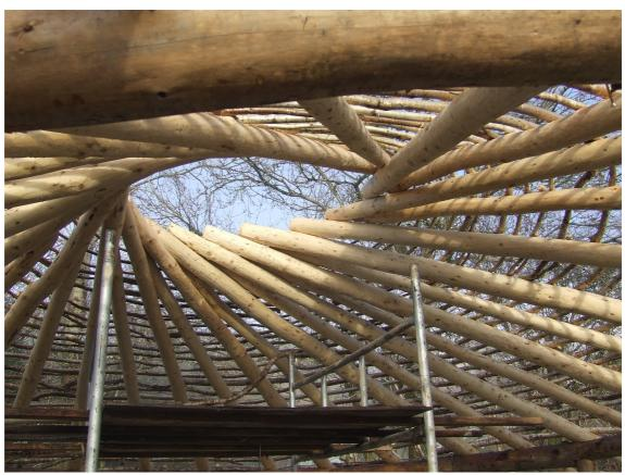
Figure 5 Photograph showing a reciprocal roof frame (c) Forde
