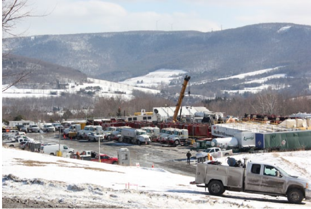
Figure 1. Fracking operation underway in northeastern Pennsylvania. Citizen Sense 2015.
