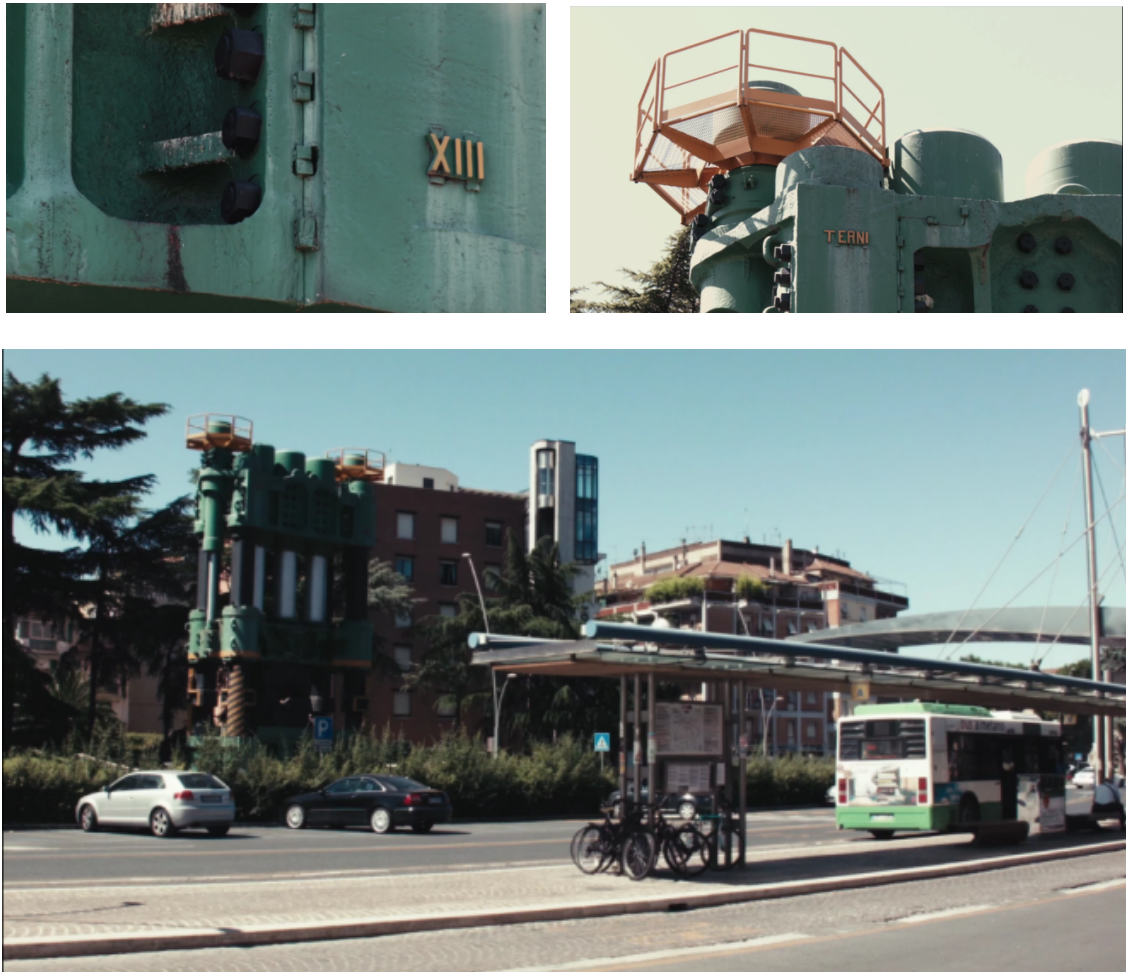
Figure 4. The 12,000-tonne press opposite the bus and train station (my photographs).
