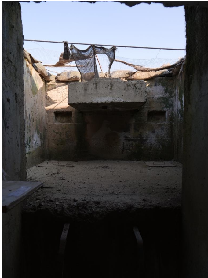
Inside the berm / tank trap.
