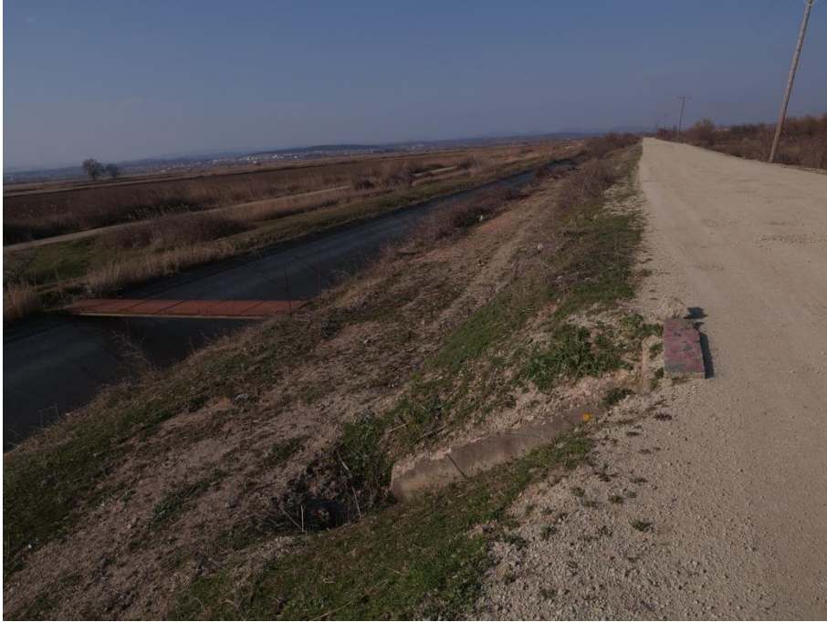
Irrigation works at the Delta near Feres.
