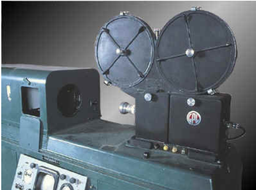
2.2.147 35mm cinema camera used to reconstruct the images received from the Lunar Orbiters on the ground in the Earth Stations
