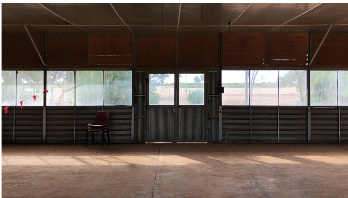
[FW 2.14] Burns, David. Maralinga Airfield Terminal V . 2018.
