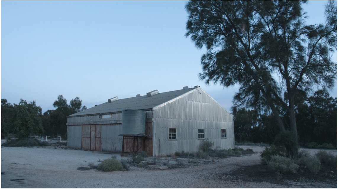
[FW 2.5] Burns, David. Old Fire Station (Maralinga Village) . 2018.
