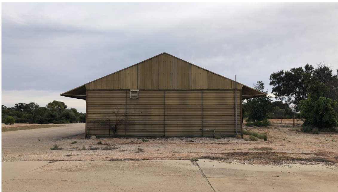
[FW 2.13] Burns, David. Maralinga Airfield Terminal IV . 2018.
