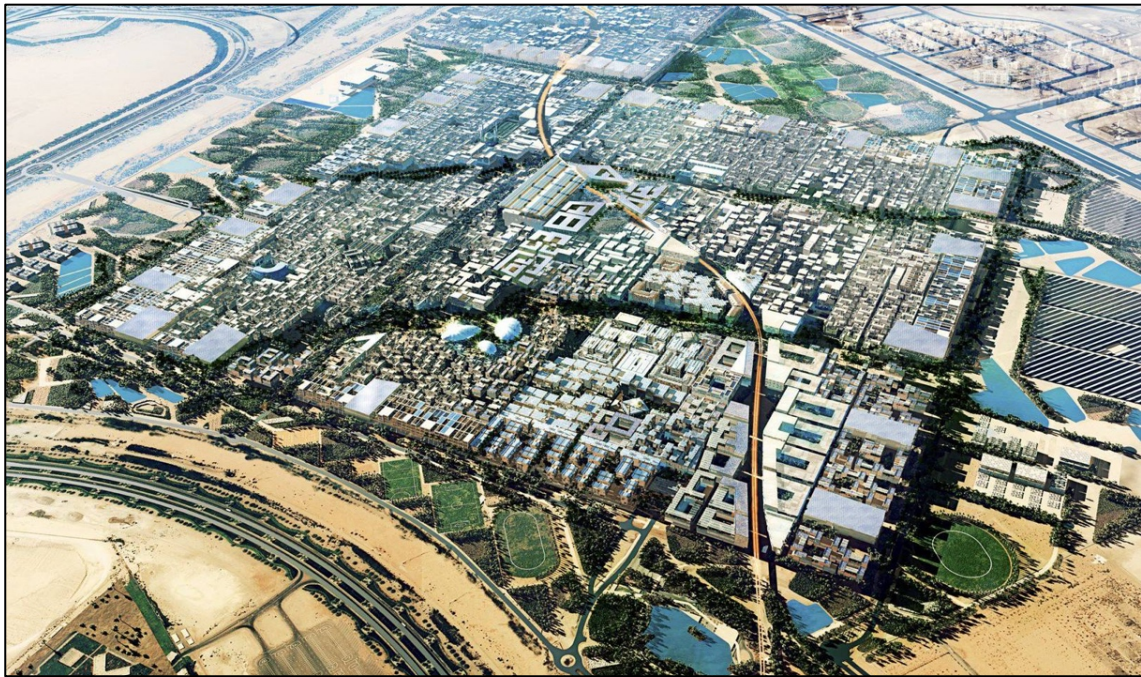
Fig. 5—Rendered aerial view of Masdar Smart City, United Arab Emirates (Foster & Partners, 2008)
