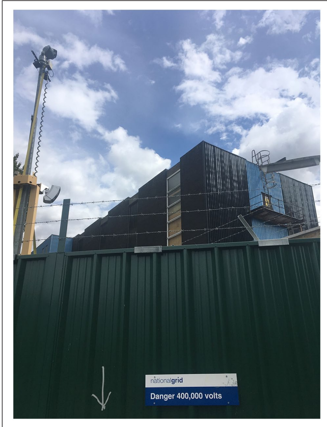
Figure 3. Following the London Power Tunnels: Hackney Substation Headhouse (photo: Laura Henneke, August 2018).
