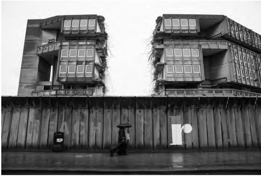
Figure 8.1 West block of Robin Hood Gardens under demolition. (Kois Miah, December 2017)
