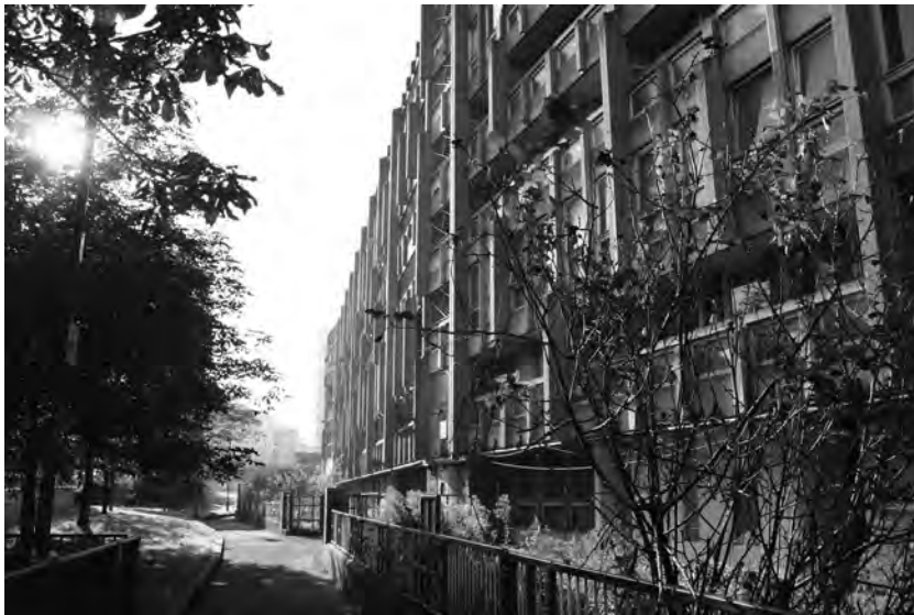
Figure 6.7 Mullions as sun-responsive forms, on the west-block garden façade. (Nicholas Thoburn, October 2015)
