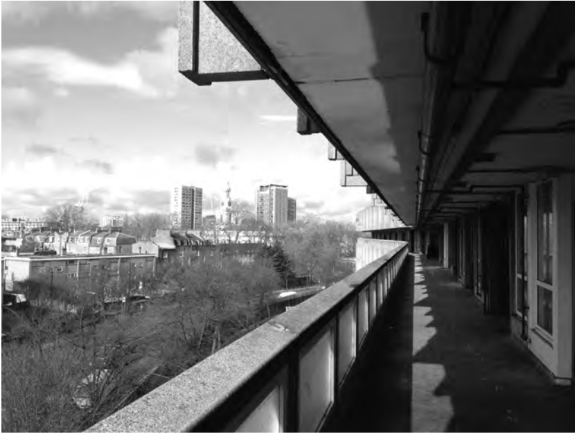
Figure 3.1 Street in the sky, west block, looking north. (Nicholas Thoburn, October 2014)
