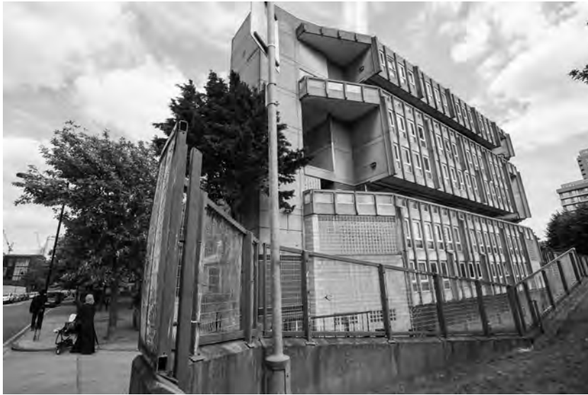
Figure 6.2 Northern “tail” of the west block, in-situ concrete in the guise of system-build. (Kois Miah, June 2015)
