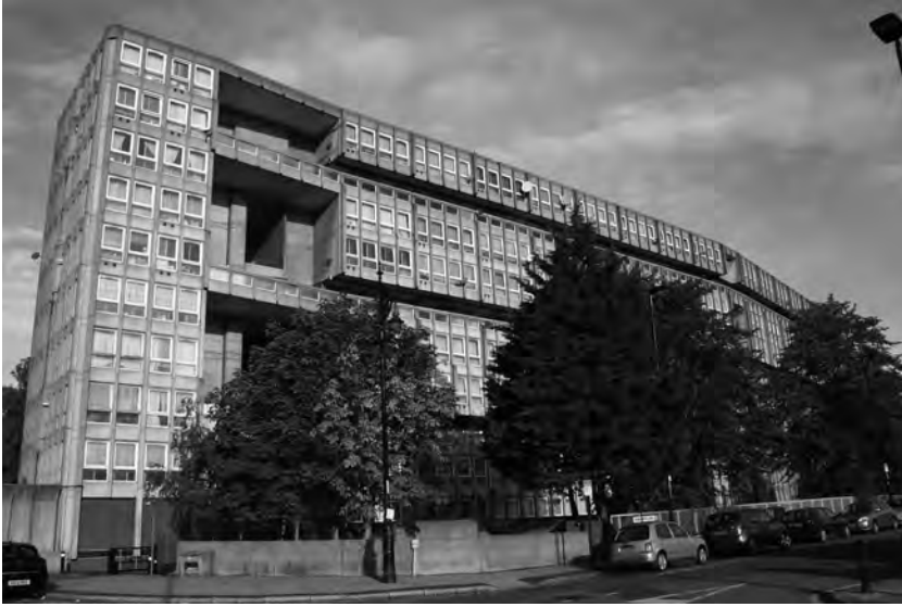
Figure 3.4 Exterior façade and southern “head” of the east block, showing the impressed bands of the three street decks and the southern lift lobbies. (Nicholas Thoburn, August 2017)
