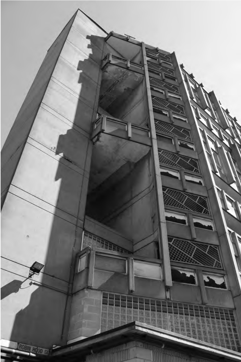
Figure 6.4 Lift-tower tail of the east block. (Nicholas Thoburn, October 2014)
