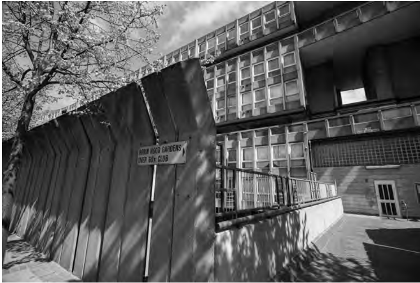
Figure 4.10 Acoustic boundary wall along Cotton Street, at the entrance to the west block. (Kois Miah, April 2015)
